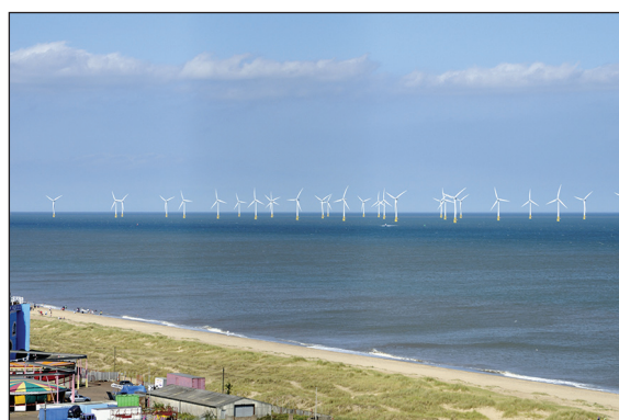
Offshore wind farm
